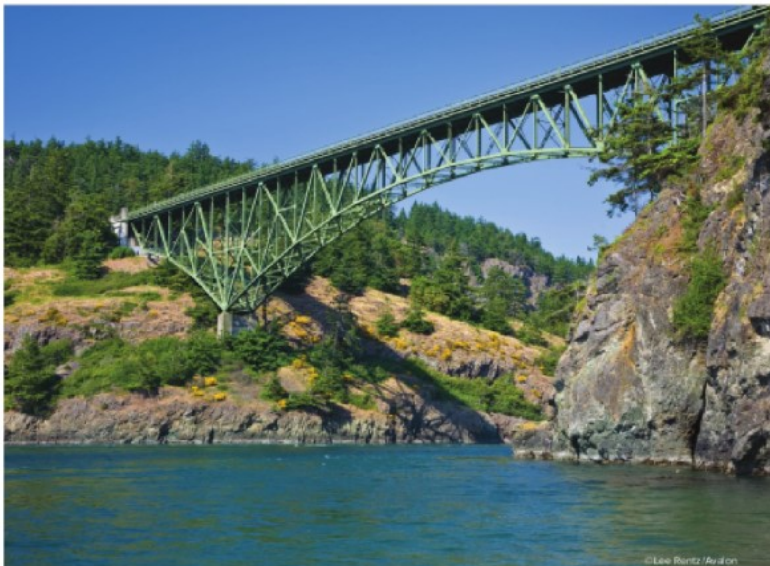
Deception Pass Bridge
